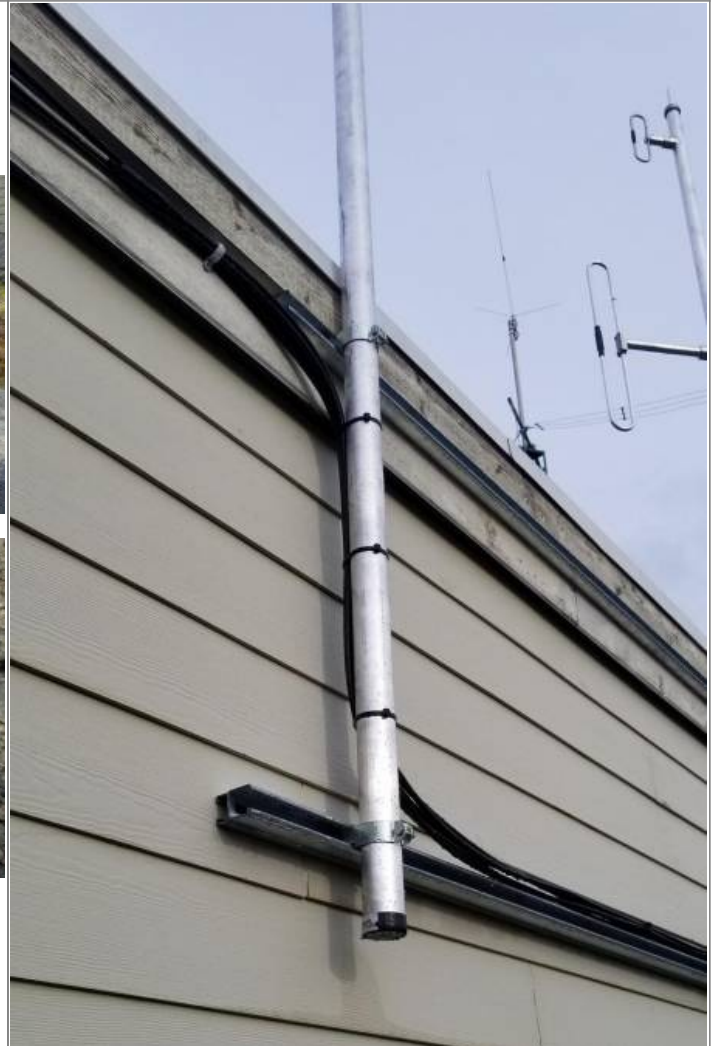
Wall mounted using Unistrut channel.
