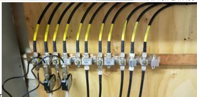
All new LMR400 feed lines tidied up and rerouted
