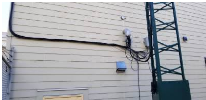
All new LMR400 feed lines tidied up and rerouted
