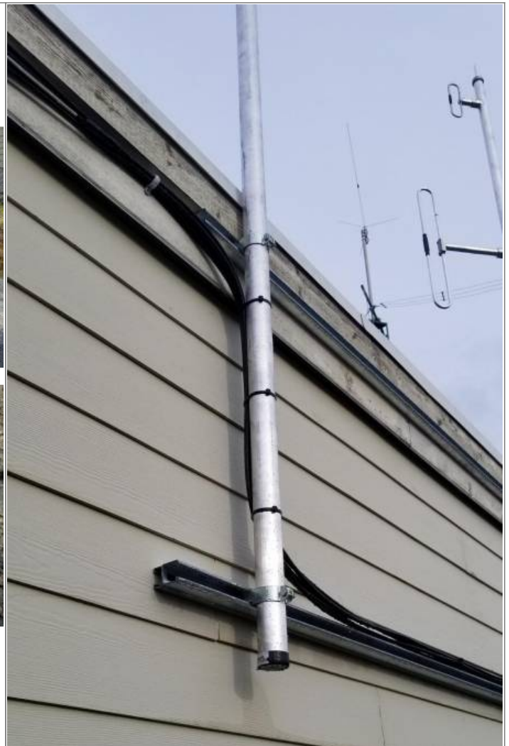
Wall mounted using Unistrut channel
