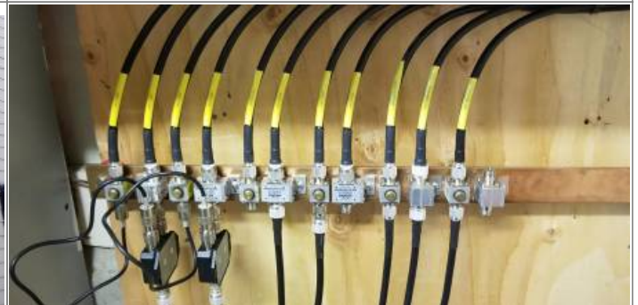
Busbar and Polyphaser/Alpha Delta surge suppression - Duplexes still to be added
