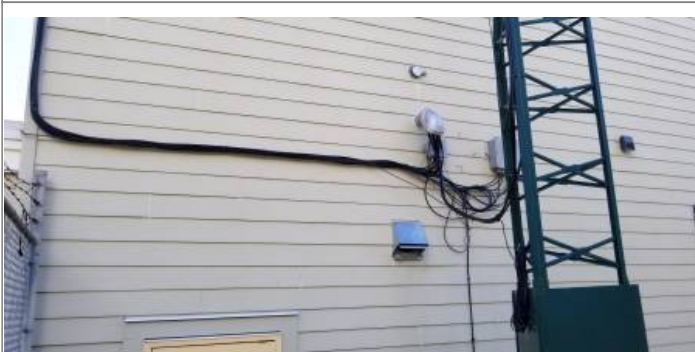
All new LMR400 feed lines tidied up and rerouted to central busbar
