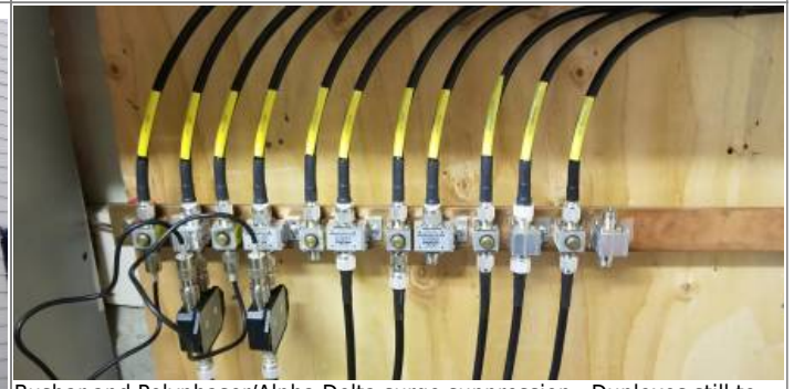
Busbar and Polyphaser/Alpha Delta surge suppression - Duplexes still to be added
