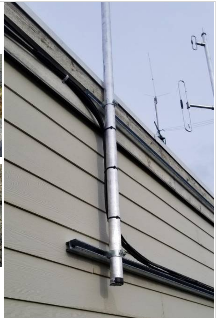
Wall mounted using Unistrut channel
