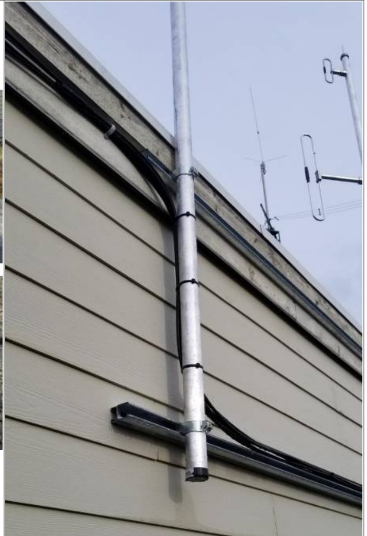
Wall mounted using Unistrut channel
