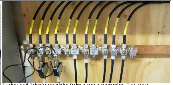
Busbar and Polyphaser/Alpha Delta surge suppression. Two more duplexers still to be added
