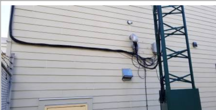
All new LMR400 feed lines tidied up and rerouted to central busbar.
