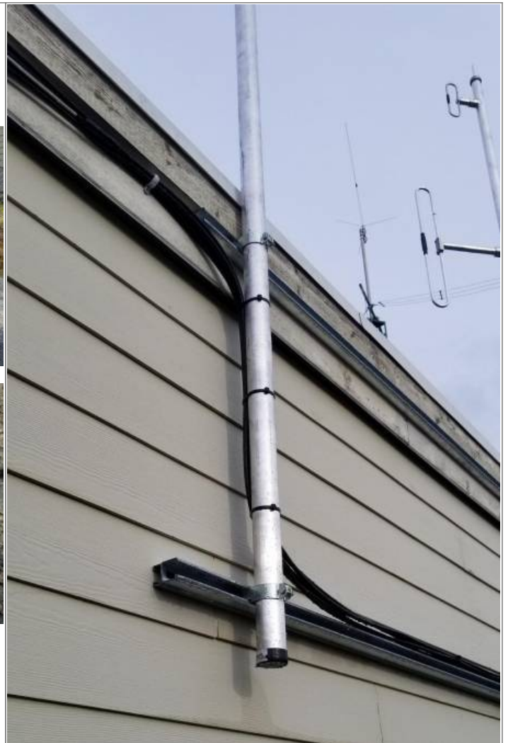
Wall mounted using Unistrut channel.
