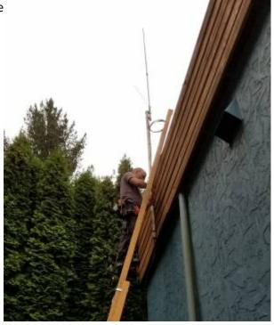
The next phase will be to run power from the comm's closet out to the top, install a grounded bus bar with a coax lightening protector, and move the repeater.
