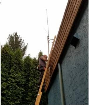
The next phase will be to run power from the comm's closet out to the top, install a grounded bus bar with a coax lightening protector, and move the repeater. Until then, the repeater is still operational at VE7HZF's place on 442.650 MHz + T100.
