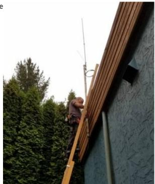
The next phase will be to run power from the comm's closet out to the top, install a grounded bus bar with a coax lightening protector, and move the repeater. Until then, the repeater is still operational on 442.650 MHz + T100.
