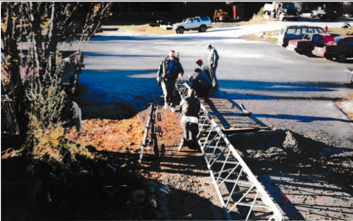
Still more bolting.
