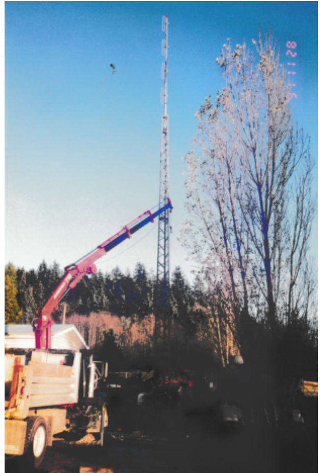
Tower is up
