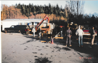
The crane ready to pull
