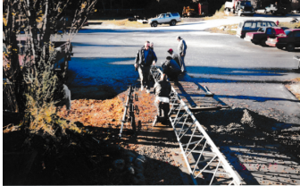
Still more bolting.
