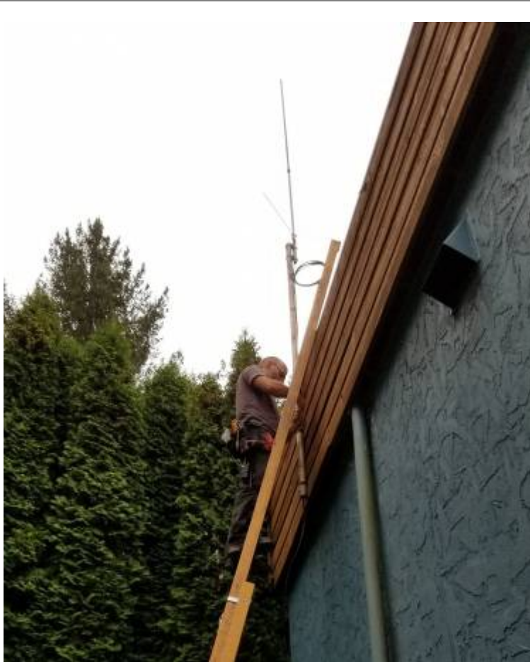
Patrick working on the antenna
