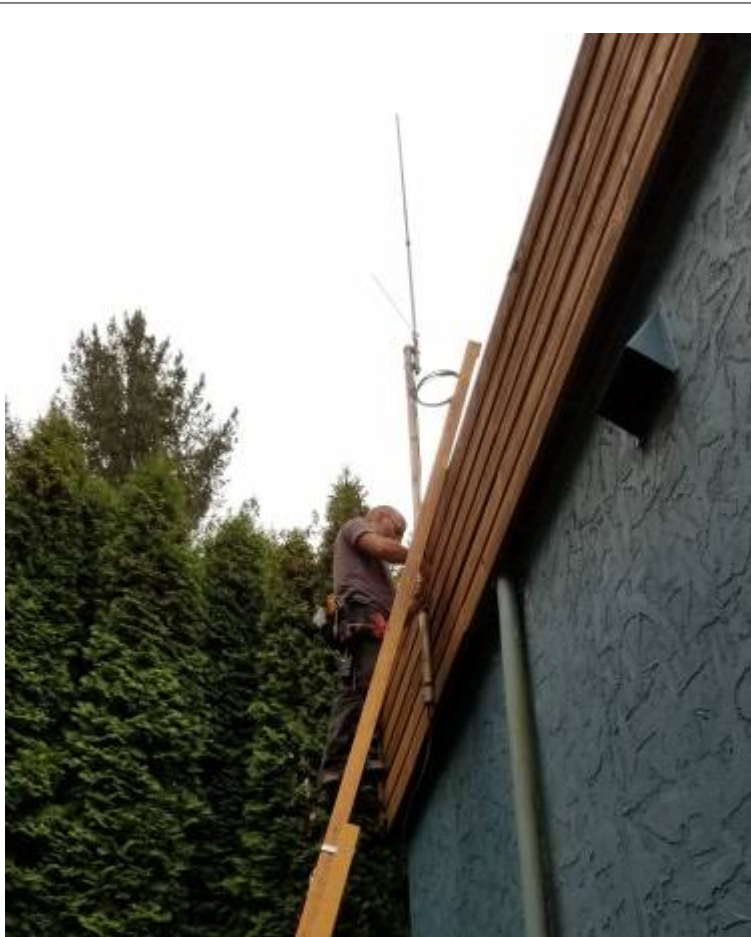
Patrick working on the antenna
