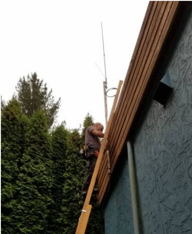
Patrick working on the antenna
