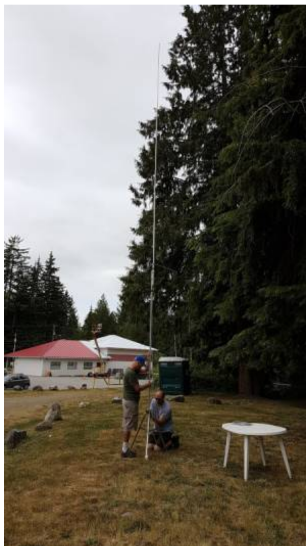
Stephen Smith (VA7SMI) holding the antenna as Robert Beaupré (VE7RBE) secures the bolts.
